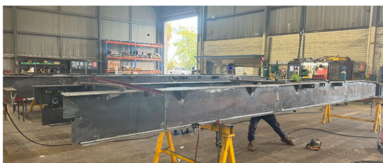
Photo of Trailer Frame Under Construction
