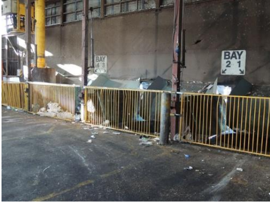
Previous Silo Tipping Area
