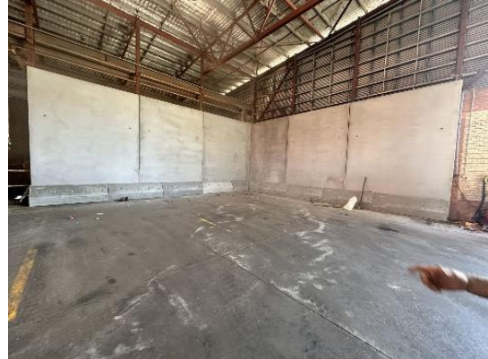
New Tipping Area
