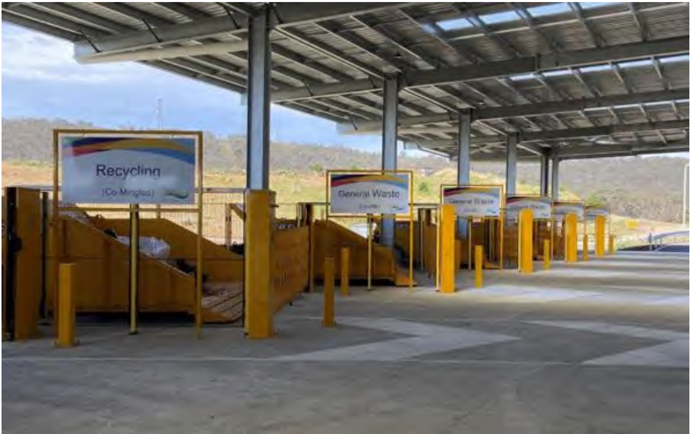
Figure 9 Safe Refuse Tipplers at Goulburn Waste Management Centre, NSW
